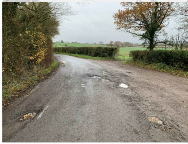
PHOTOGRAPH OF SITE ACCESS
